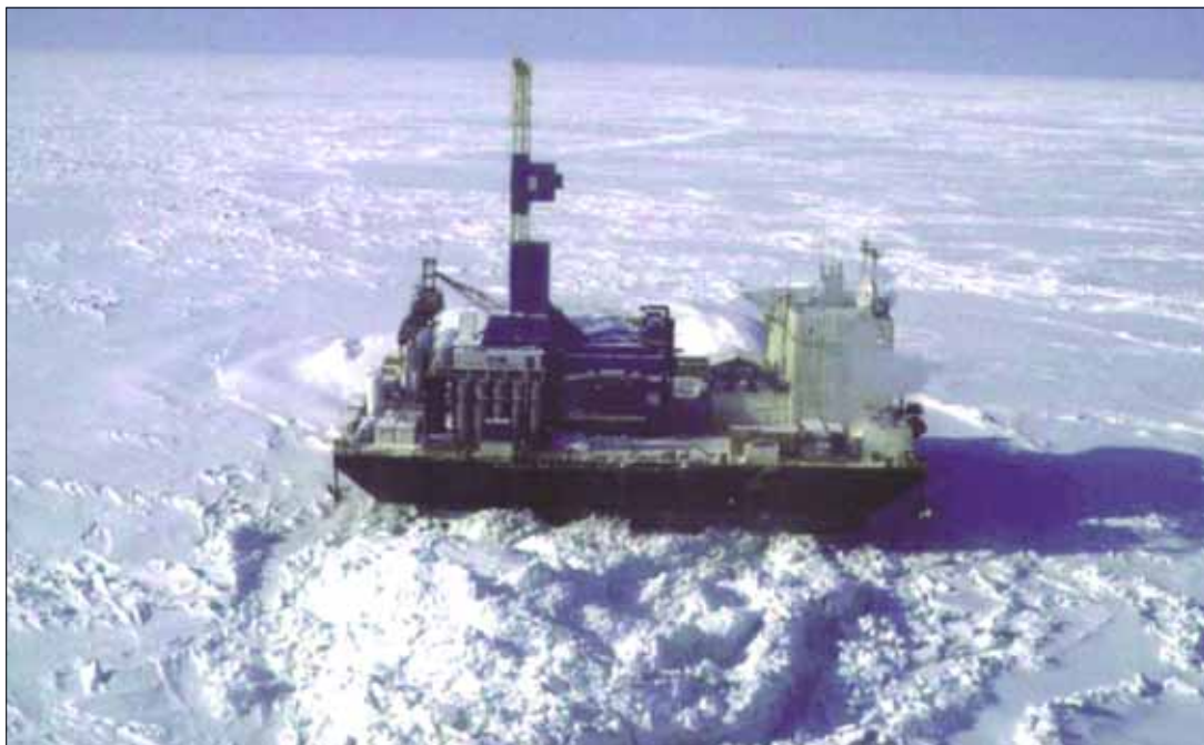
Figure 4 Concrete Island Drilling Structure (CIDS) in the Beaufort Sea, Alaska (PAME, 2002)
