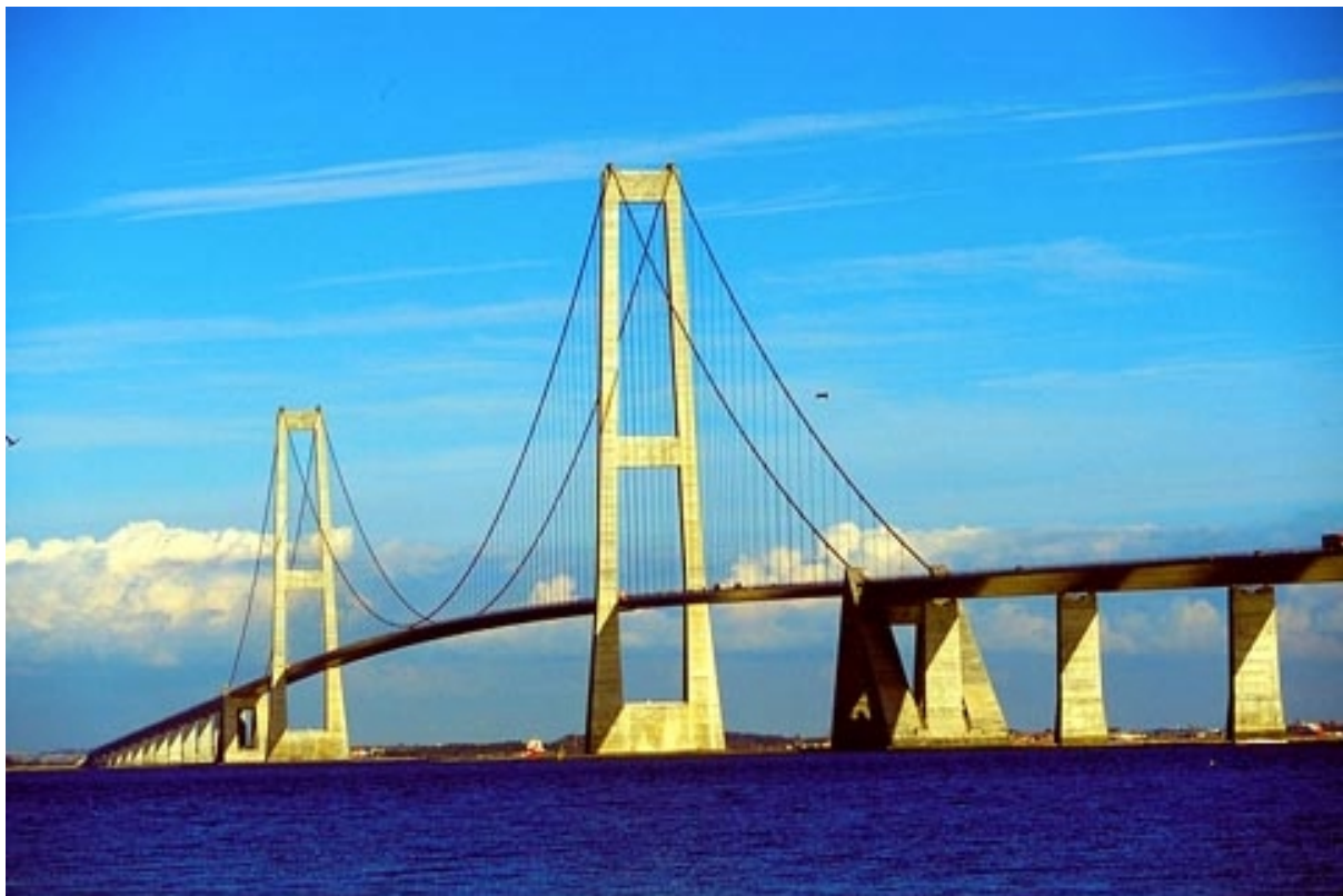
Figure 21. Great Belt Bridge (source: Great Belt a/s)
